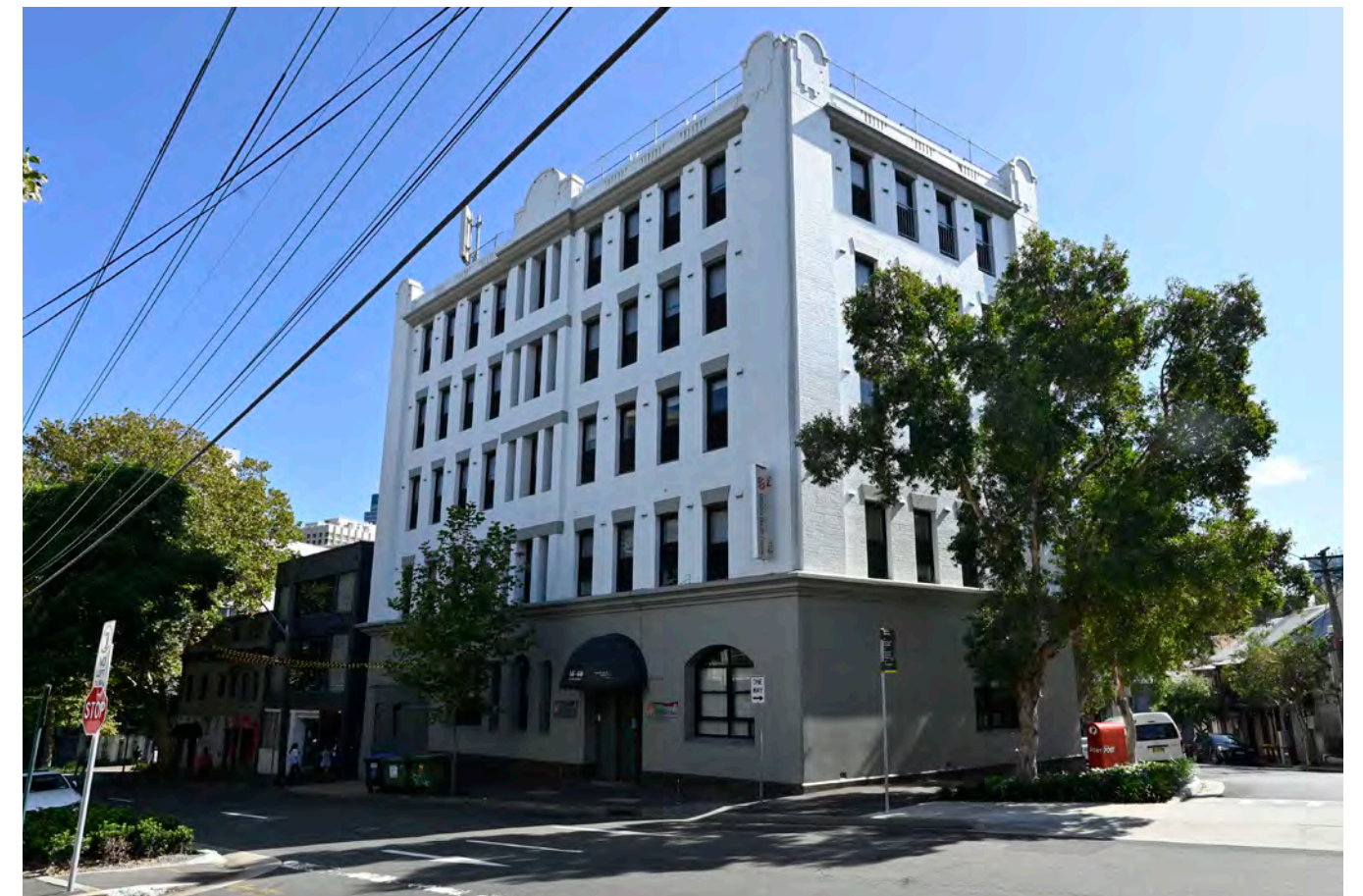
Image 1: The Salvation Army's William Booth House, located at 56 – 60 Albion Street Surry Hills
